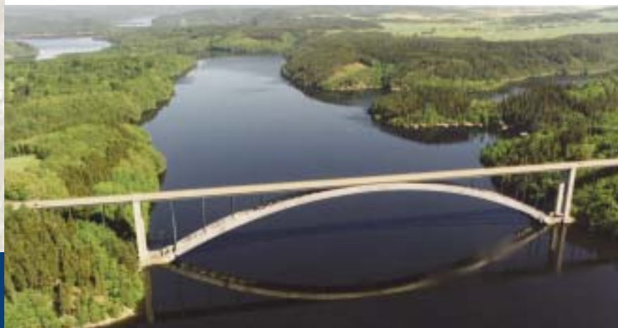
Orlík Dam and Žďákovský Bridge with the largest span of the steel arch in the Czech Republic
