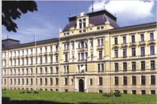
Building of the CR Ministry of Defense
