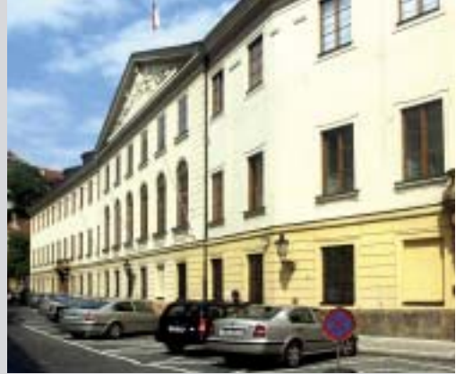
The Chamber of Deputies Building
