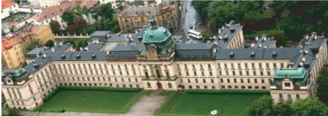
Residence of the Government of the Czech Republic
